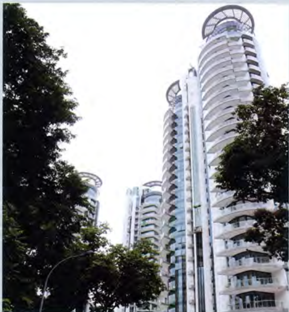
CDL's 110-unit Cliveden at Grange has recently obtained its TOP and the developer could potentially release the remaining units for sale
