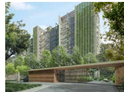
Above: JTResi has also sold units in Goodwood Residence, designed by WOHA. This development features many sustainable design initiatives, including green walls and a rainwater storage system used to irrigate the gardens.
